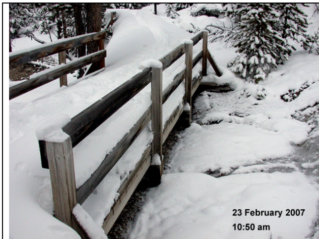
Figure 3. The boardwalk over Steamboat channel. Notice the snow and ice covering the boardwalk. Small rivulets of water upstream of the boardwalk show the extent of normal thermal erosion.
